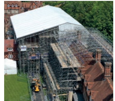
Bradfield College with asymmetric solution to its tall chimney stacks
