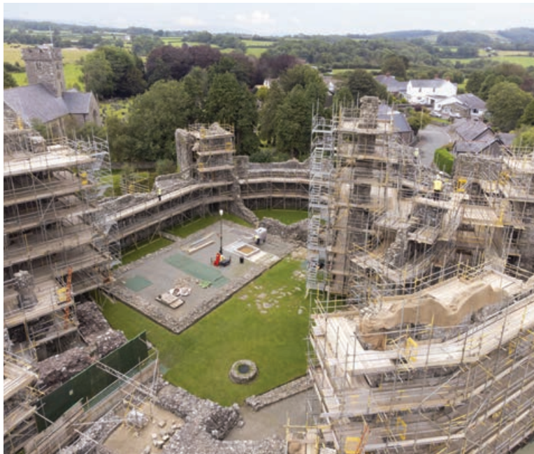
Access was needed for Coity Castle conservation work
